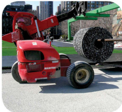
Picture 1. Rolls make for quick and easy installation
